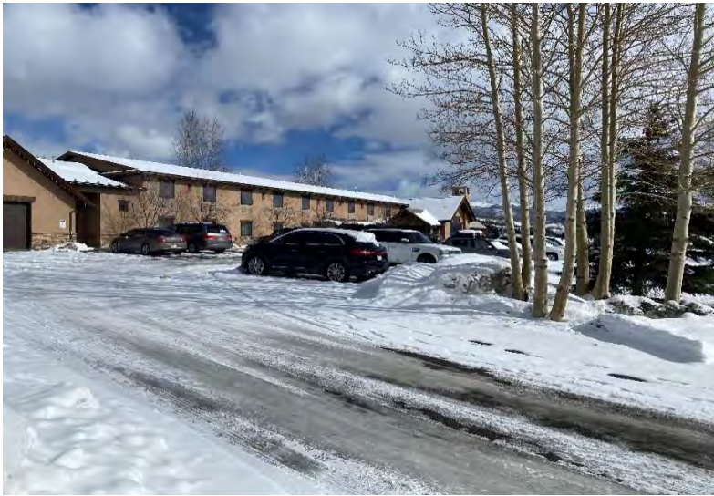
View of easterly adjoining Alpine Inn. View to the northeast.
